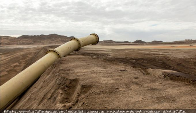
Following a review of the Tailings deposition plan, it was decided to construct a starter embankment on the north-to-north eastern side of the Tailings Storage Facility and a buttress on the western side, with the work completed towards the end of 2015. These two stability reinforcement projects will ultimately enable us to deposit tailings in an area on the facility that was previously not suitable for tailings deposition.
